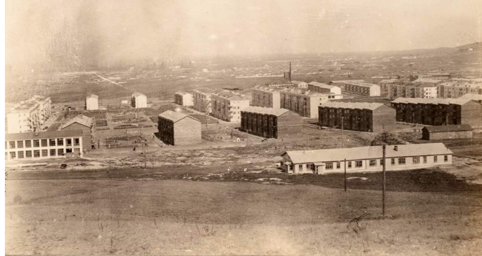
Fig. 7. Dwellings sotsgorod Magnitogorsk with at the left crèche designed by Grete Schütte-Lihotzky, 1932-35. Courtesy of Canadian Centre for Architecture, Montréal.
