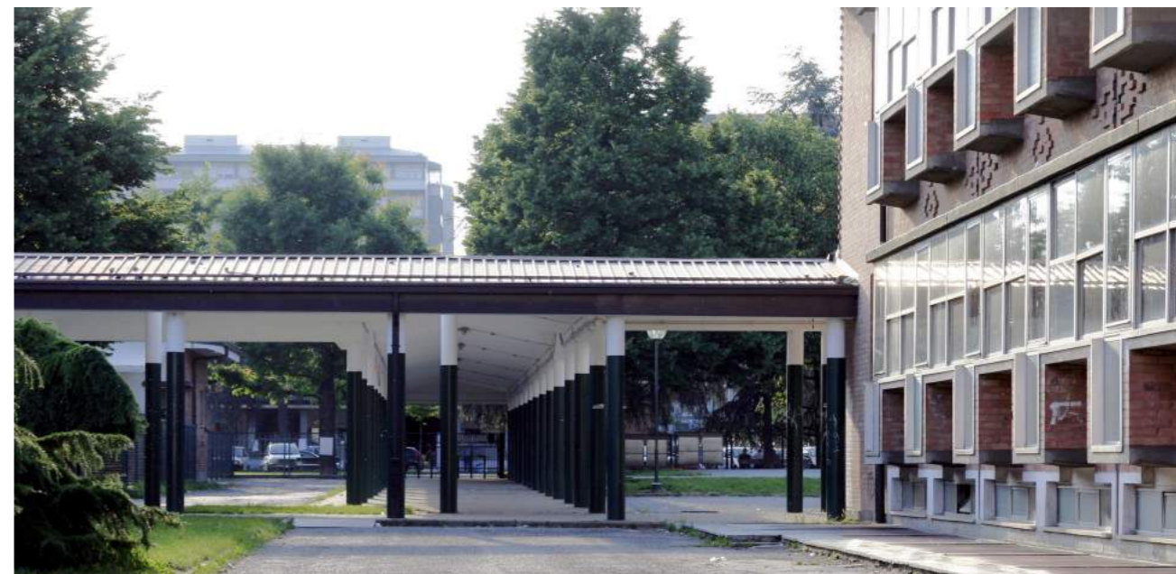
Fig. 9. Ada Bursi, School in via Duino, Turin 1969. Photo by Caterina Franchini.
